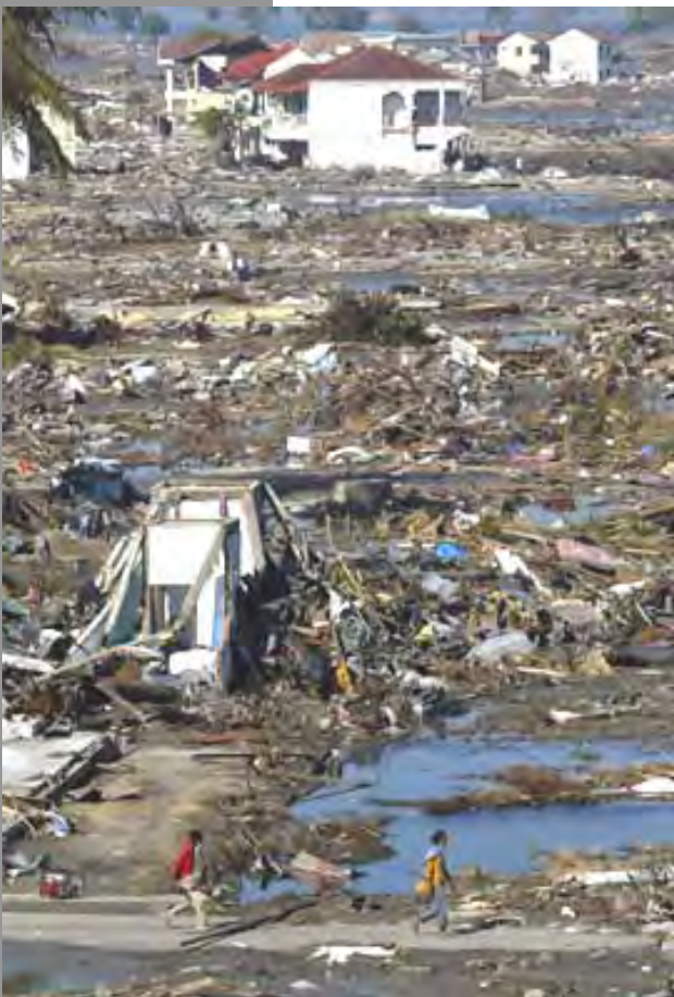
The ruins of a housing complex in the Indonesian city of Banda Aceh three days after the disaster. Photo International Federation
