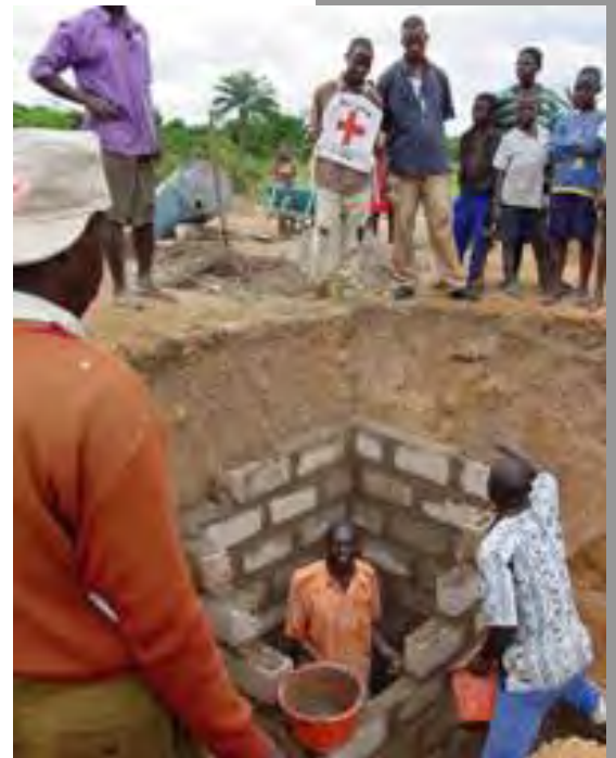
Building a latrine Photo: International Federation
